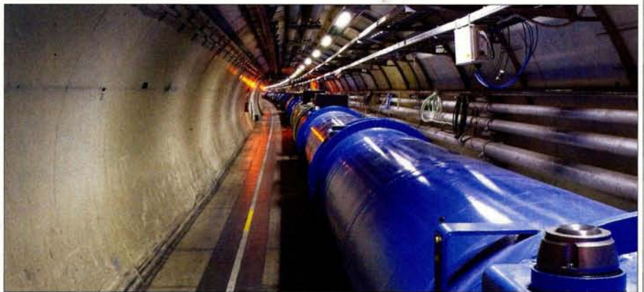
This is not an artist's impression! A long line of superconducting magnets is beginning to wend its way along the 27 km tunnel of the Large Hadron Collider.
